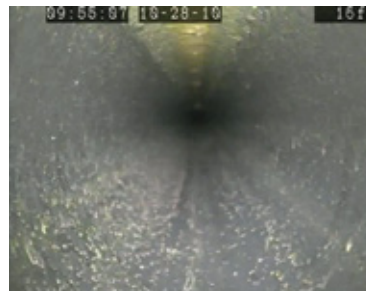
Branch line at 16ft with no corrosion, water filled with no air-water interface
