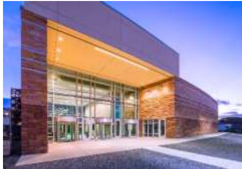
U.S. Army Pacific Command & Control Facility Fort Shafter, Hawaii
