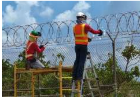
Typhoon Mawar Repair & Recovery Guam
