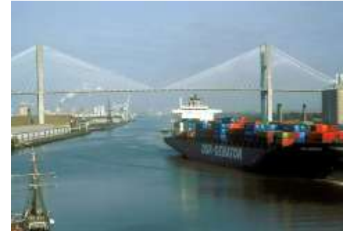
Savannah Harbor Navigation Project Savannah, Georgia
