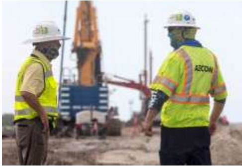
Herbert Hoover Dike Lake Okeechobee, Florida
